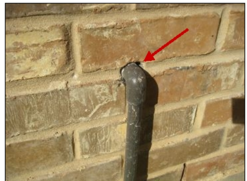
Seal sprinkler wire entry to home on right elevation
