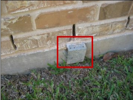
Remove mud sill anchor at the rear elevation of home
