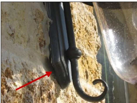
Seal around all exterior wall penetrations
