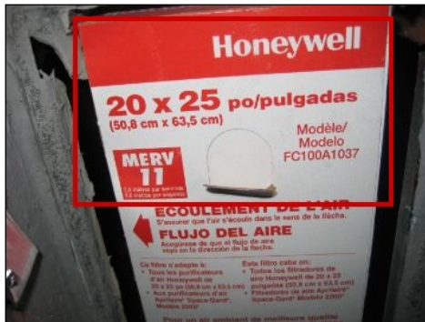
Filter size and type at plenums
