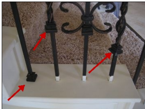
Spindles boots not secure
