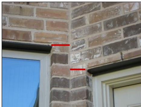
Lintels should have minimum 4" bearing
